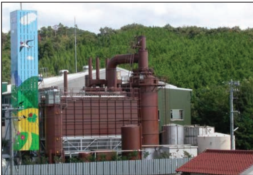
FIGURE 3. This is a general view of the filter plant and direct cooling chamber at Honshu I. The ceramic filter plant can be seen center left in the plant. To the right of the filter plant is the direct cooling chamber and to the left the exhaust stack
