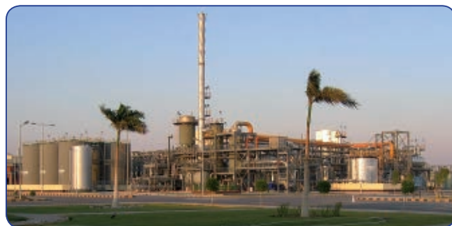
Desmet Ballestra 450 t/d sulfuric acid plant in Egypt
